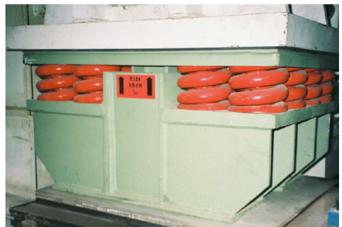
KTI spring supports with a bearing capacity of 1,600 kN
