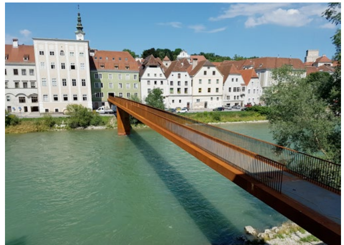
Footbridge over the Enns with two TMDs' after installation
