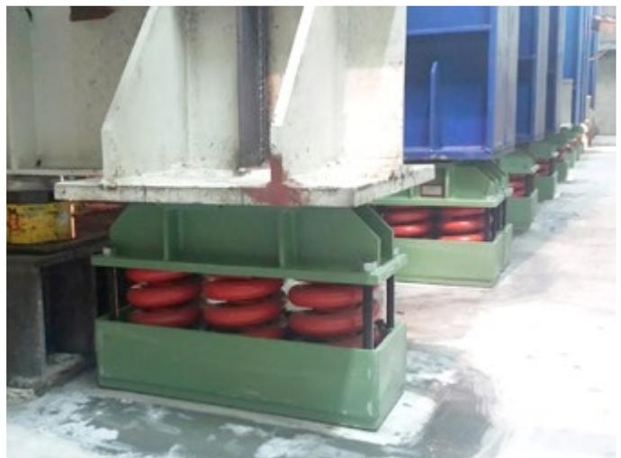
**Spring Isolators for suspension of a test stand**
