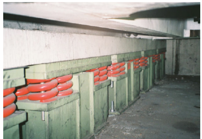
KTI spring supports for convincing emission protection
