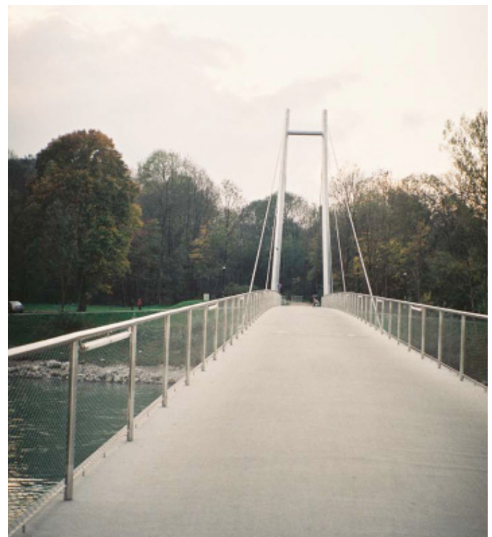
Cable-stayed bridge over the Salzach near Salzburg, Austria
